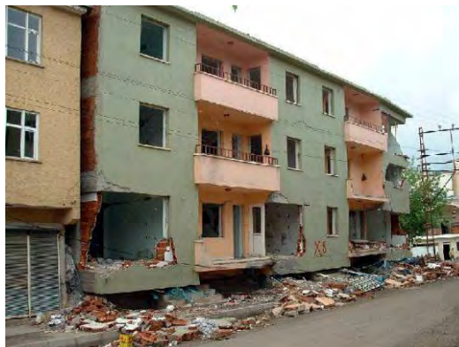
Gambar 1. Soft-storey - Gempa Bingol, Turki 2003
